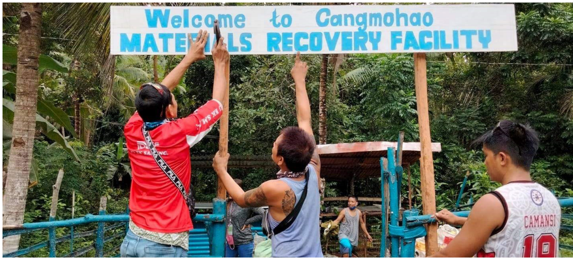
Constructing a materials recovery facility
