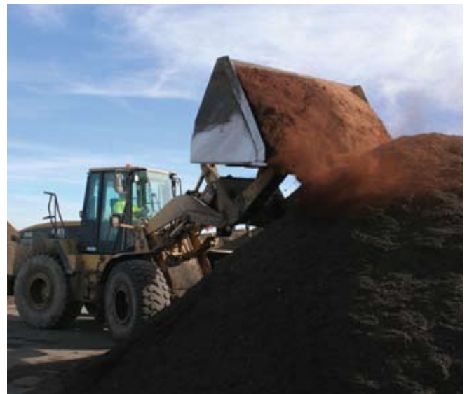
The blending pad at Jepson Prairie Organics, a modern compost facility used by San Francisco. (photo: Larry Strong, courtesy of Recology)
